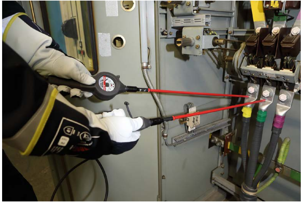
Fig. A 5-22 Determining a voltage-free state
