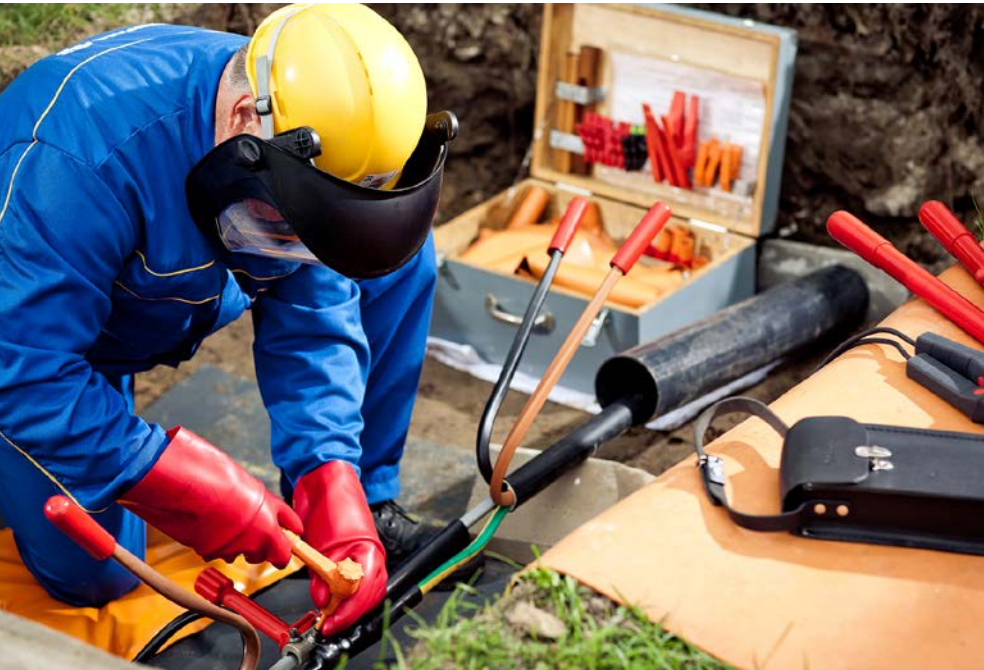
Fig. A 6-5 Installing cable sleeves: k_T = 1.9
