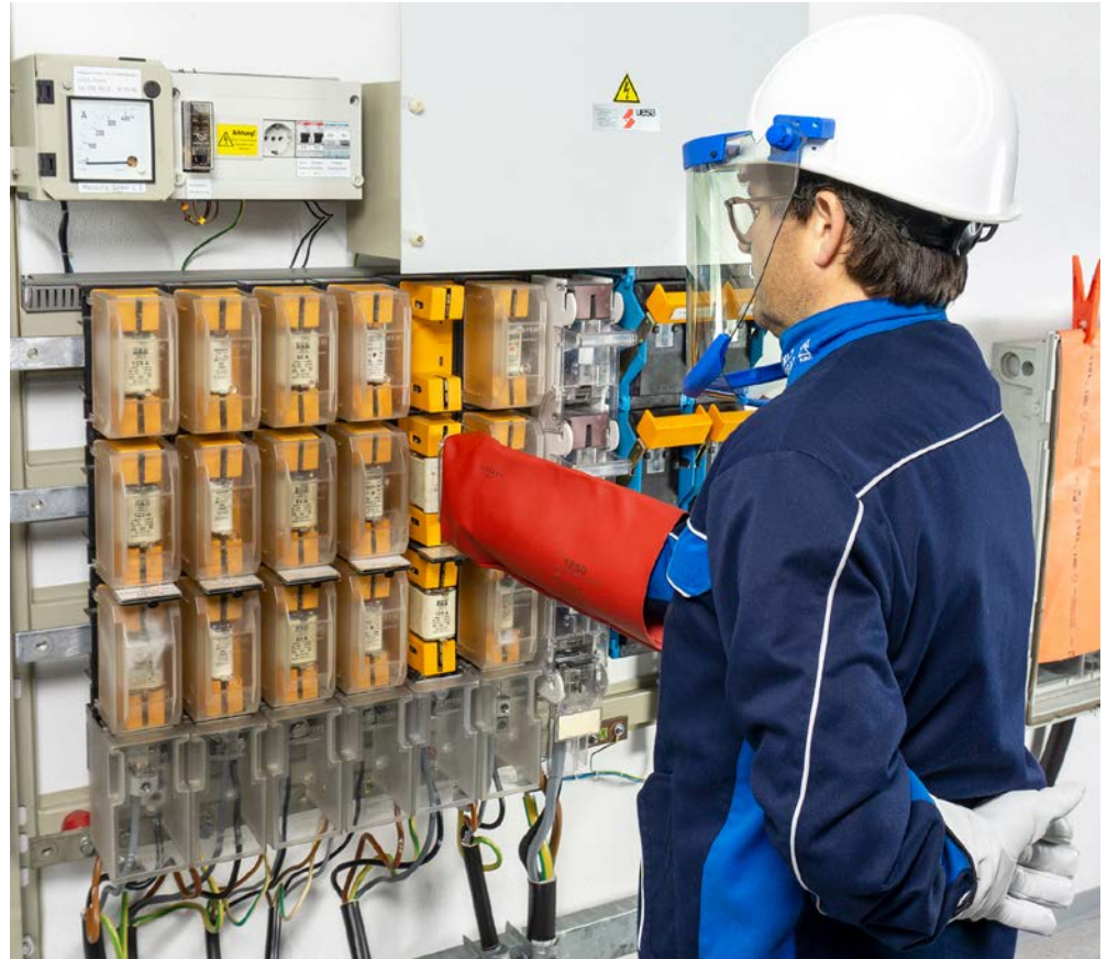
Fig. A 5-2 Working on a low voltage distribution system
