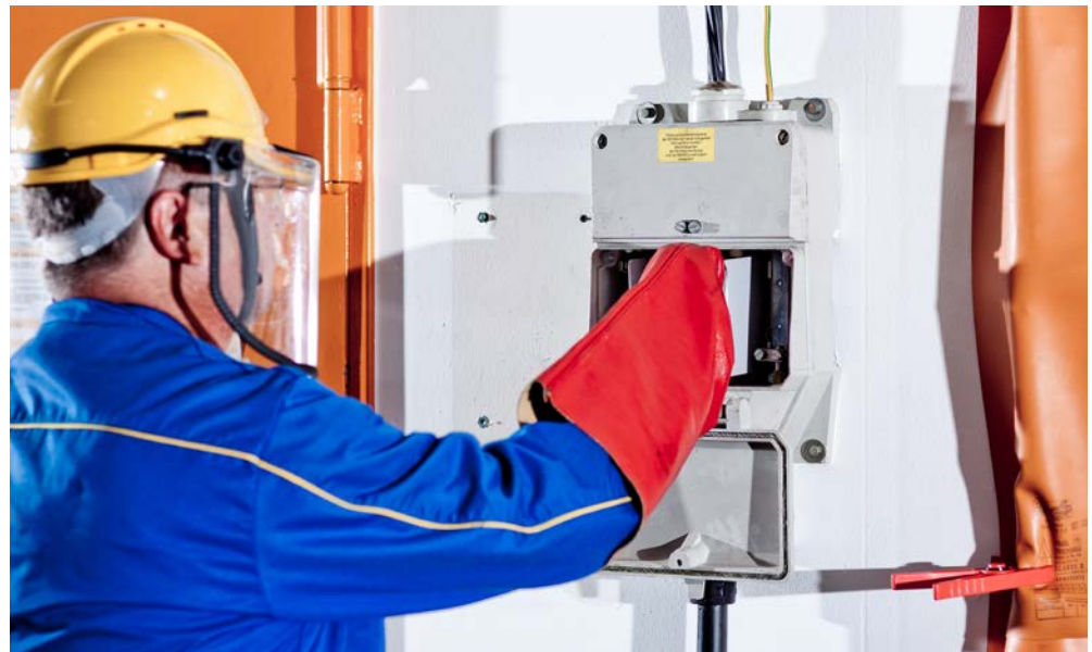
Fig. A 5-11 Removal and installation of NH fuse-links in a house junc- tion box
