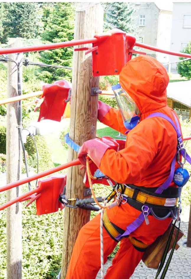
Fig. A 6-6 Working on an electricity pole: k_T = 2.4
