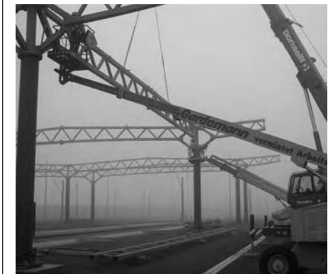
Fig. 9: pre-assembly on the ground and installation with an aerial work platform
