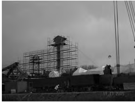
Fig. 4: Working and safety scaffolds
