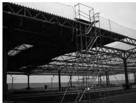
Fig. 13: Freestanding stair towers
