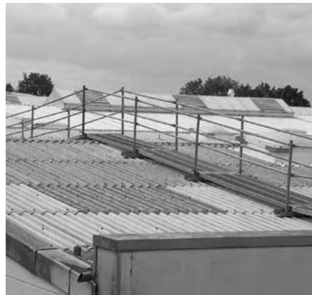
Fig. 15: covering which distributes the load
