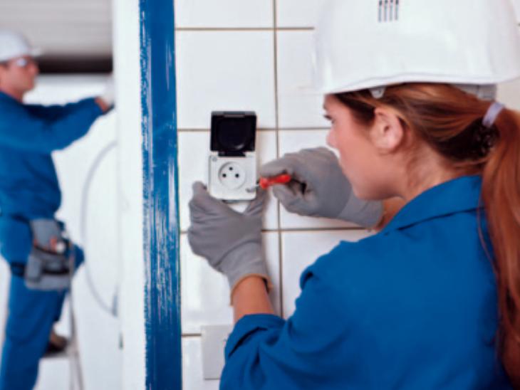
Mounting of a power plug in a sanitary
