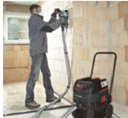
Pictures 1 and 2: Examples of harmonised systems: Wall grinders and angle grinders with conversion kits for wall grinders with a dust-removing unit of Dust Class M
